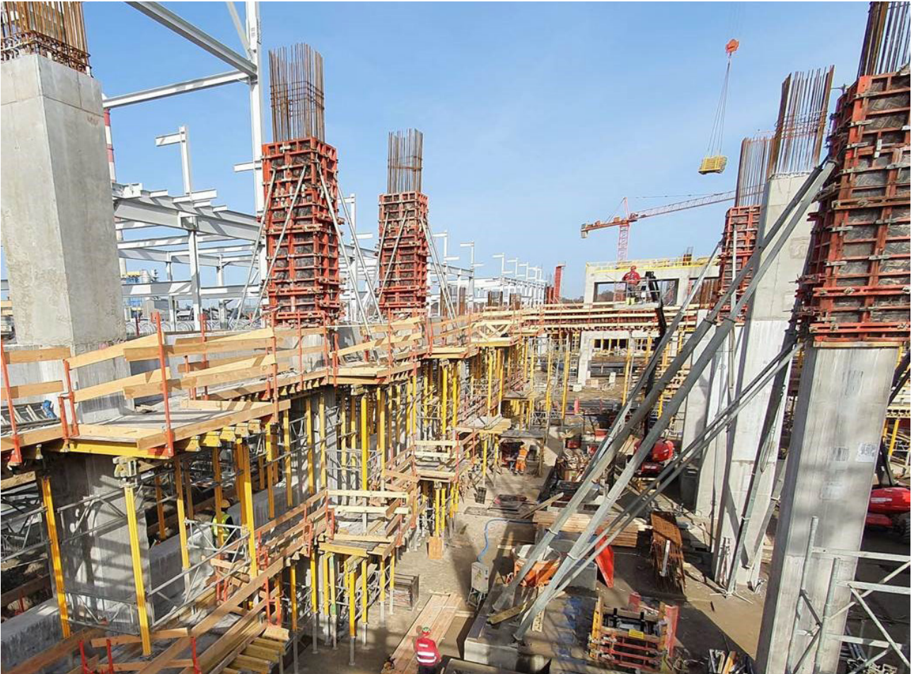
Construction of the Polimery Police complex, Police, Poland
